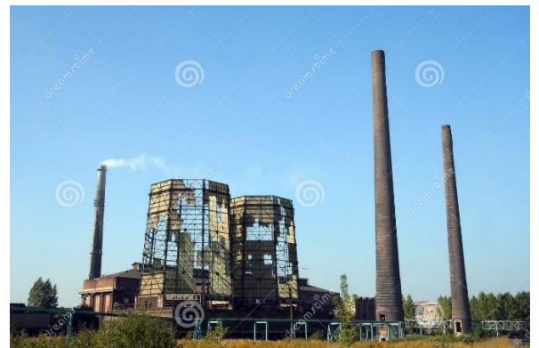
Figure 14 Destroyed Cooling Towers (Consider the Cartoon Theme)
